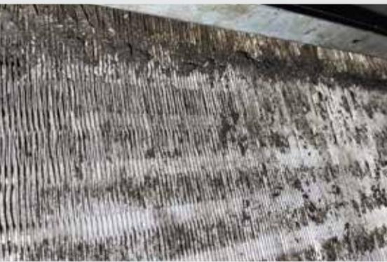
Figure 2: A common coil cleaning attempt to restore HVAC performance
